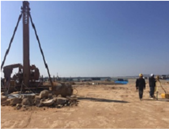
The construction site of the processing factory
